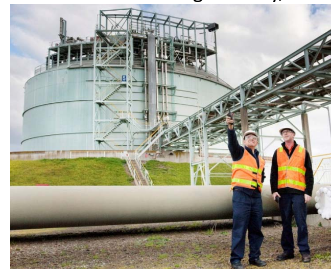
Dandenong LNG Storage Facility, Vic
